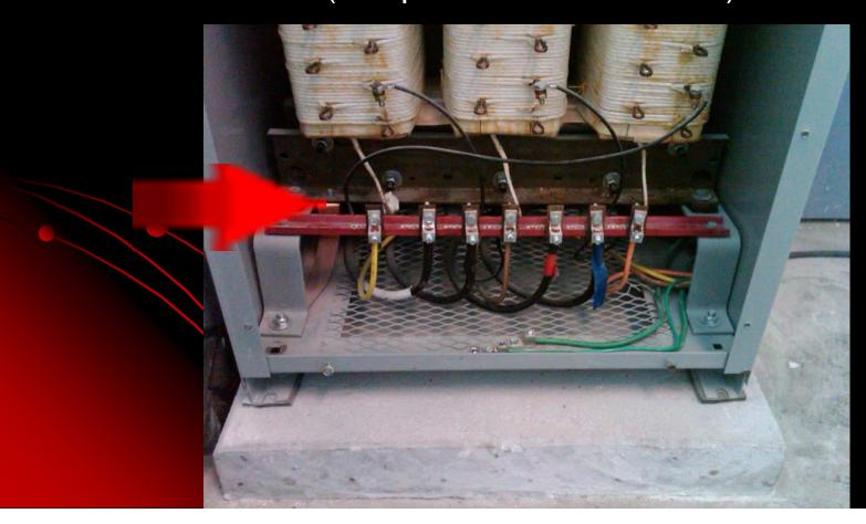
Wiring (XO Missing Bonding Jumper)
