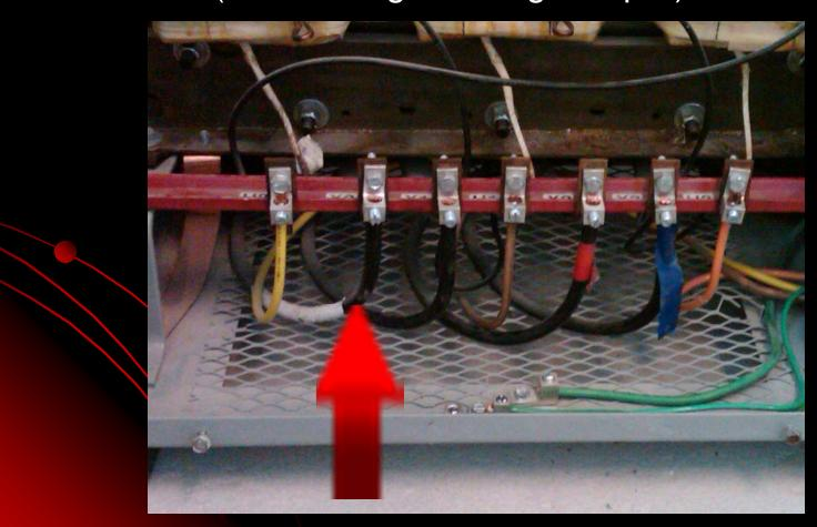
Wiring (XO Missing Bonding Jumper)
