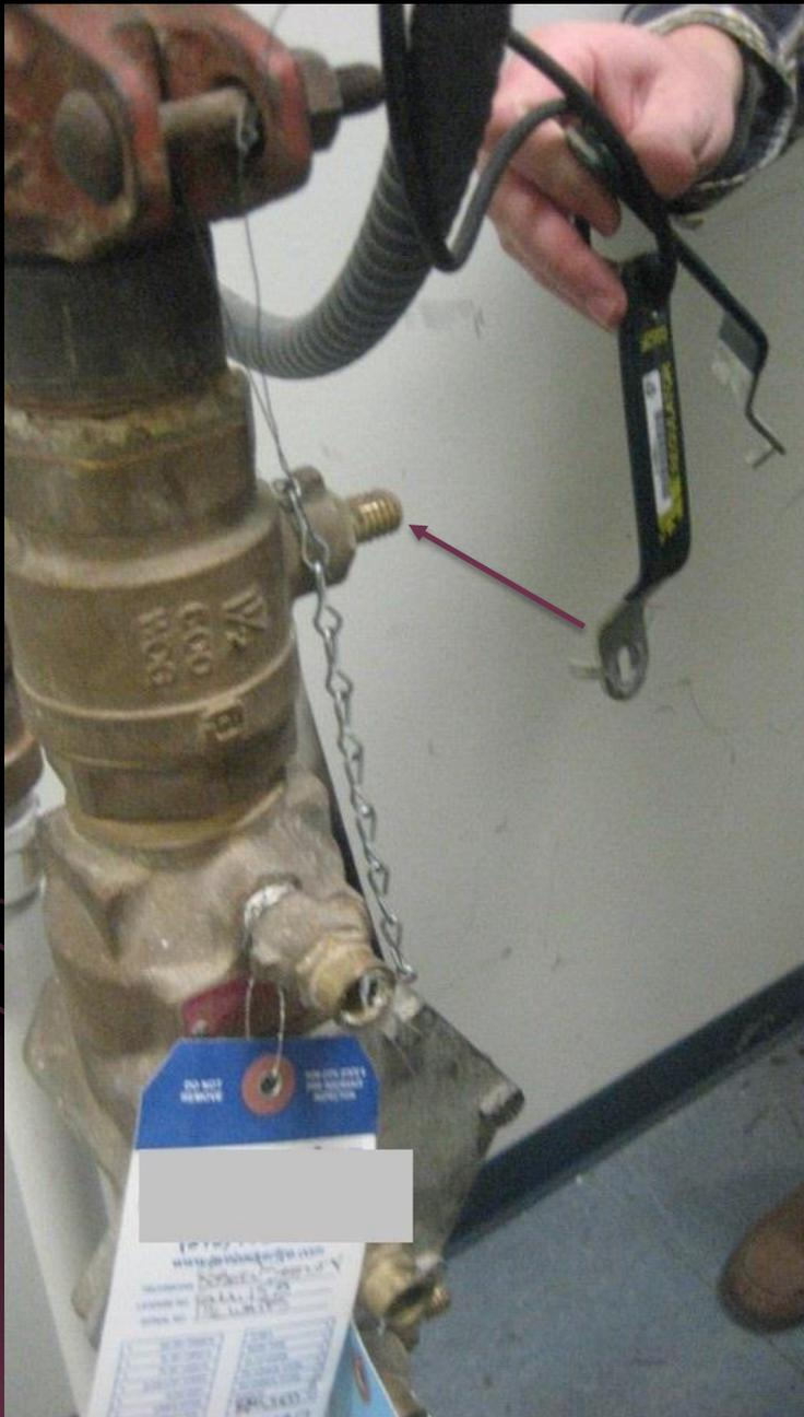
To eliminate breaking & replacing the electronic cable, the handles were removed at annual testing.
