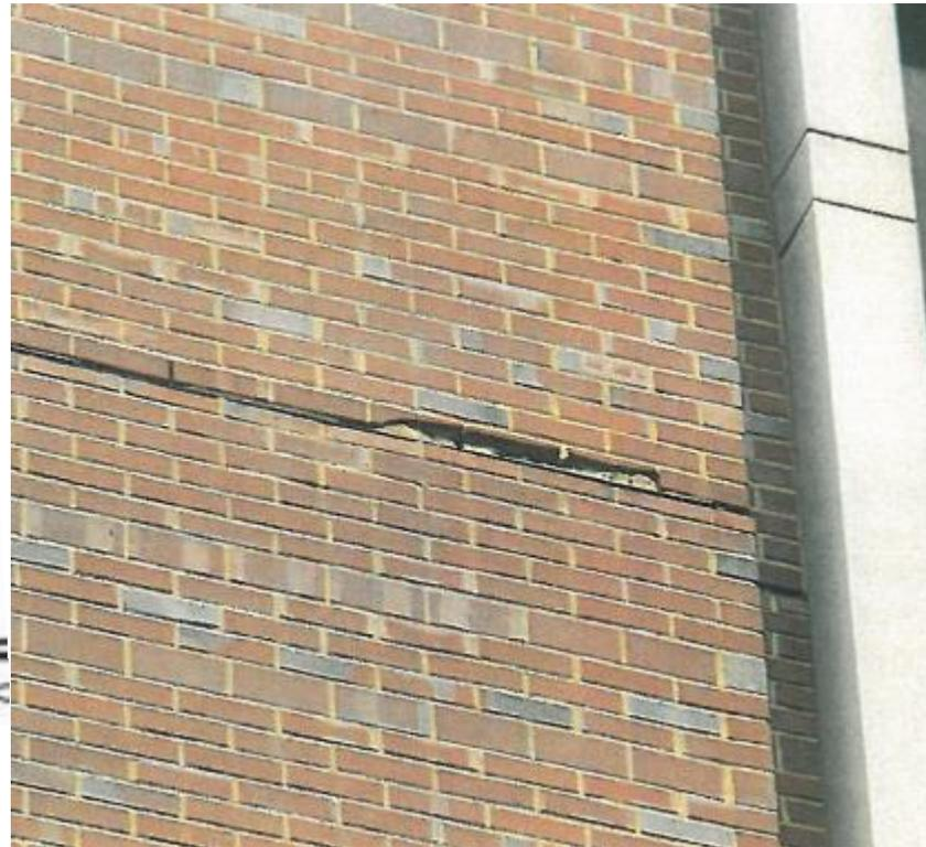
Site fabricated brick falls away from building due to freezing
