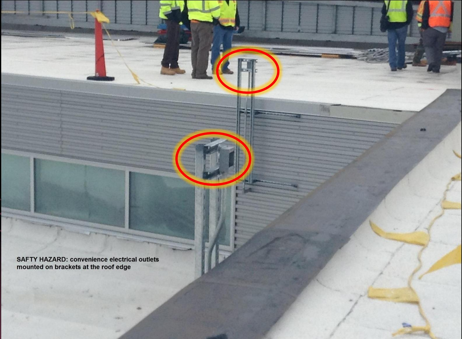
**SAFETY HAZARD:** convenience electrical outlets mounted on brackets at the roof edge
