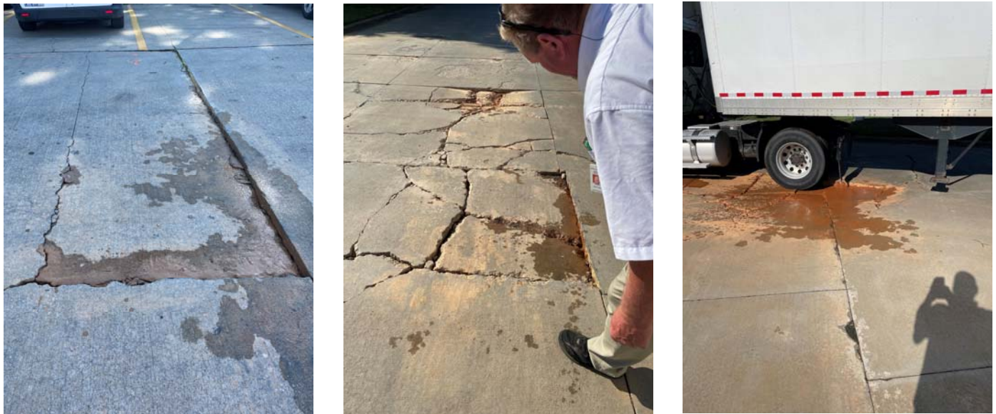
Figure 1 – Existing Loading Area and Entrance photos
