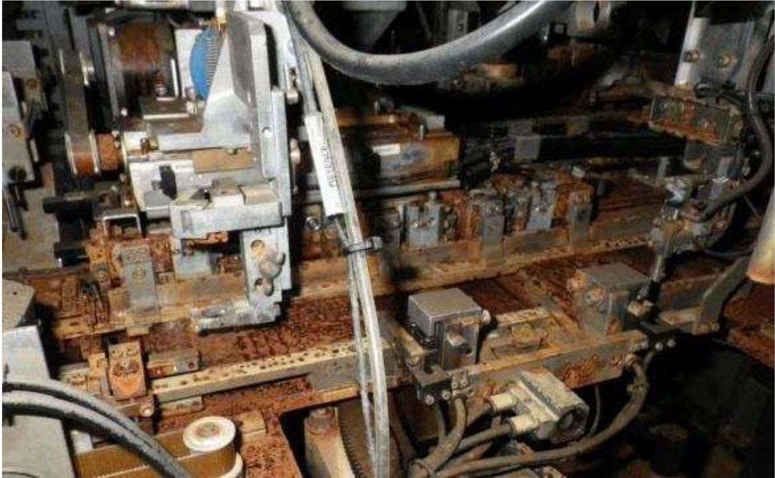
Corrosion can affect protective equipment clearing time including “no trip” failure mode
