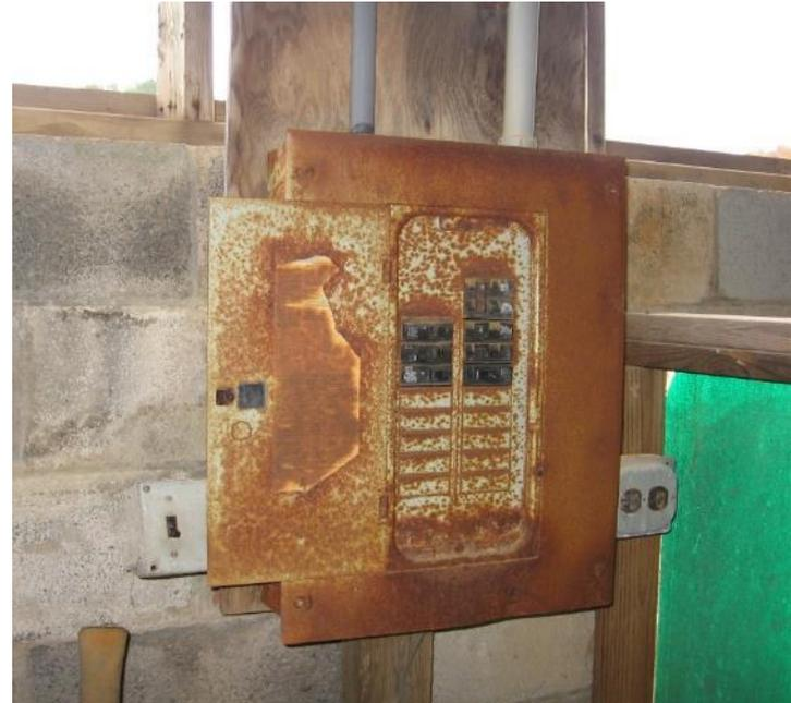
Corrosion is *accelerated* by increased concentration of contaminants, elevated temperature and high humidity.
