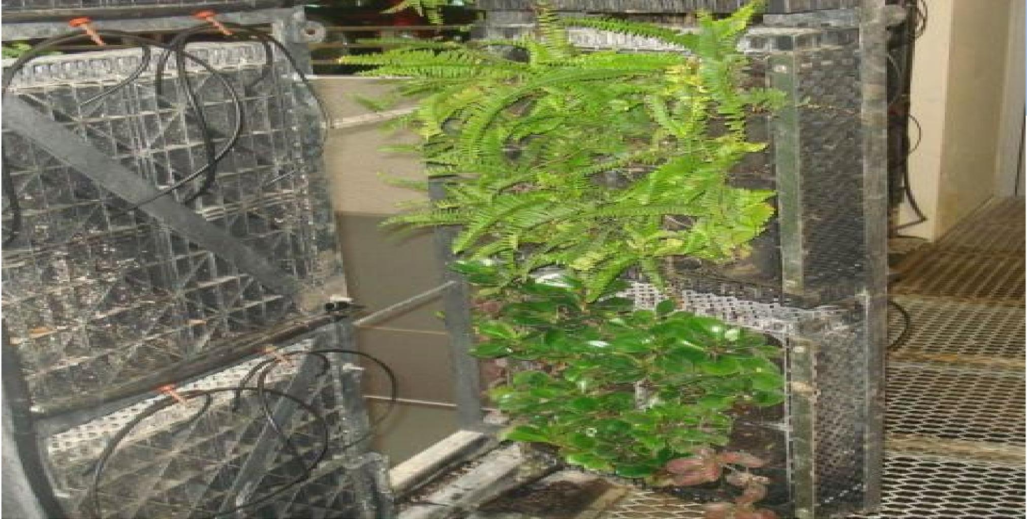
“French doors” allow the greenery to come to the worker. The camouflaged guardrail is aesthetically pleasing and is a passive control that allows workers to safely maintain and replace the vegetation without much planning.
